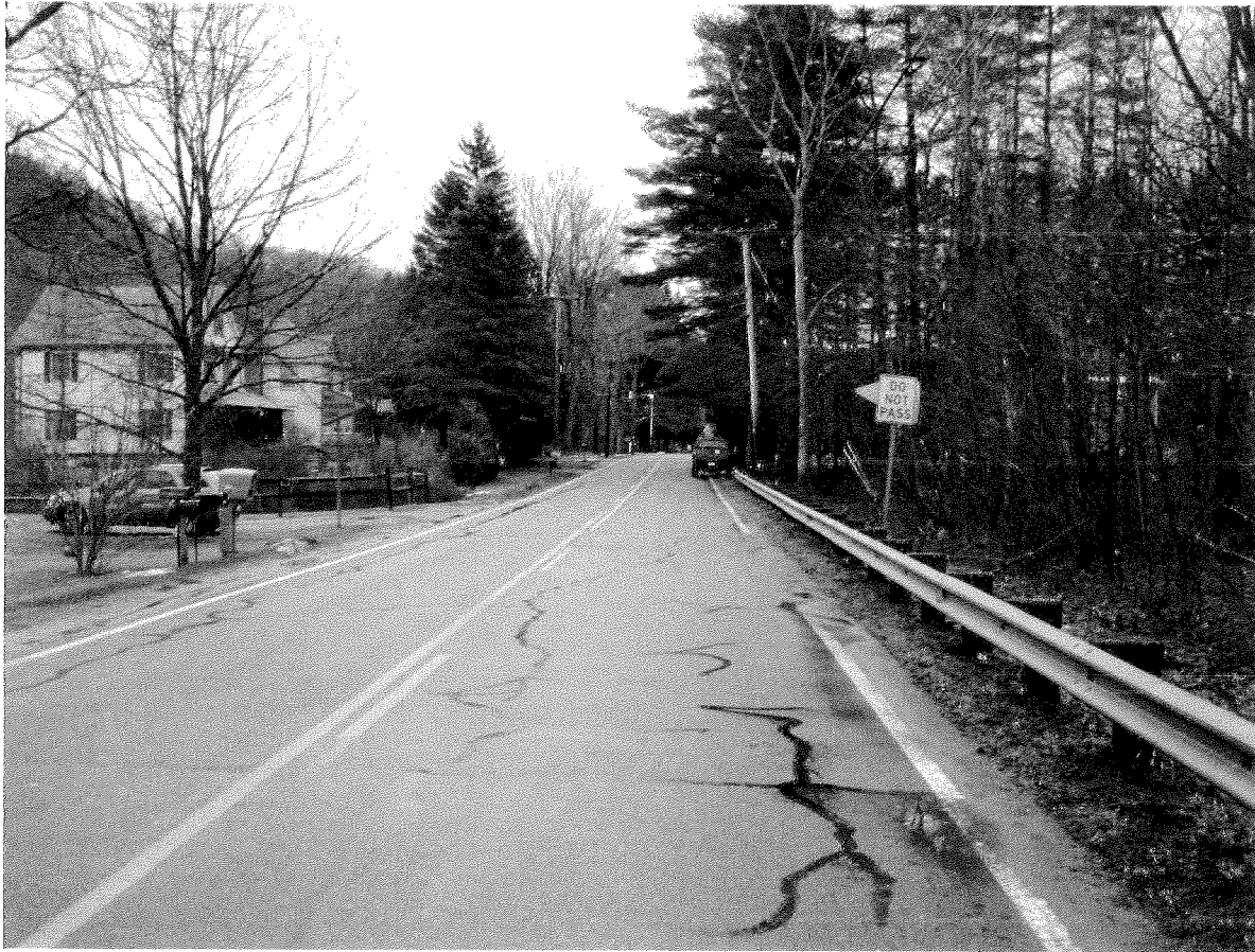
Rte. 183 / Park Street Looking South
